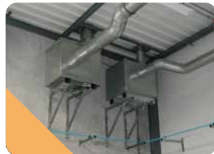
Caissons sur chaises Acoustic enclosure in wall
